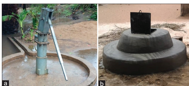
Figure-2: Some wells from which water samples were collected. (a) Borehole. (b) Concrete cased well.
